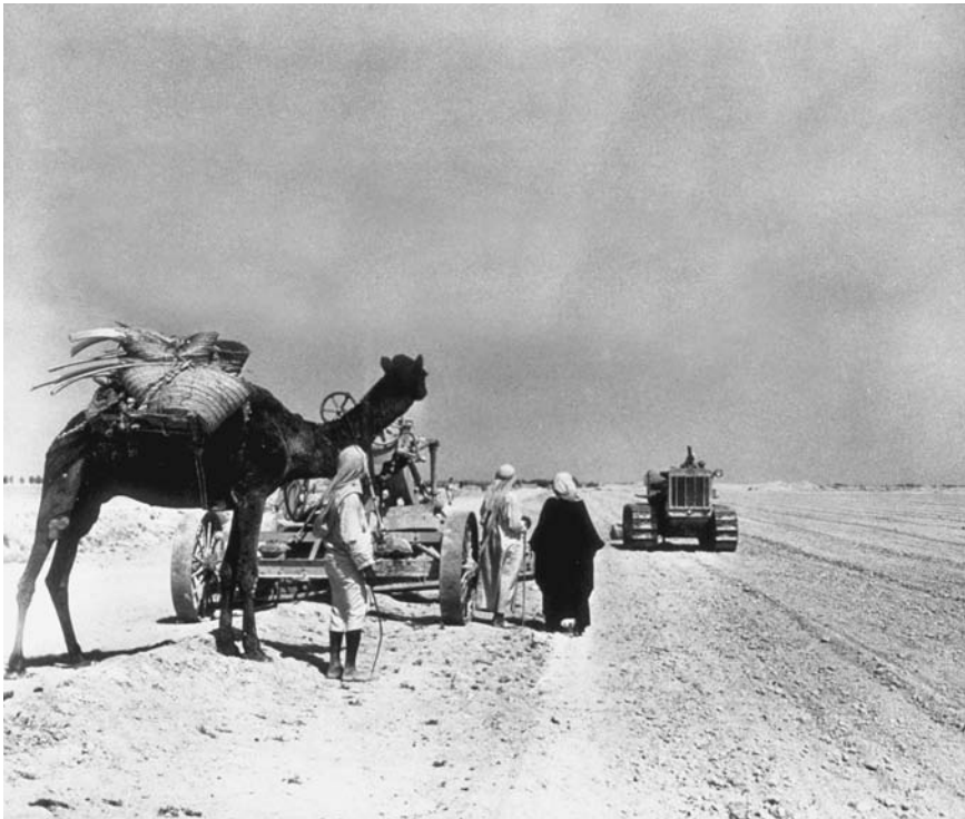
Confrontations between old and new became increasingly common after the discovery of oil. This 1947 photograph shows a Bedouin and his camel crossing paths with modern machines in the midst of road building near Hufuf. (Courtesy of Robert Y. Richie/Aramco World/PADIA)
