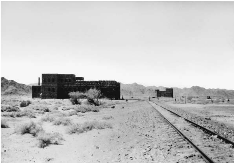
The train stations of the Hijaz Railway were built so they could double as fortresses. Note the height of the first-floor windows above the ground. (Courtesy of the Fine Arts Library, Harvard College Library)
