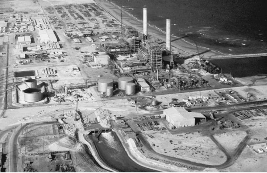
The Ghazlan steam-powered generator plant was a major project designed and implemented as part of a five-year development plan. (Courtesy of B. H. Moody/Aramco World/PADIA)
